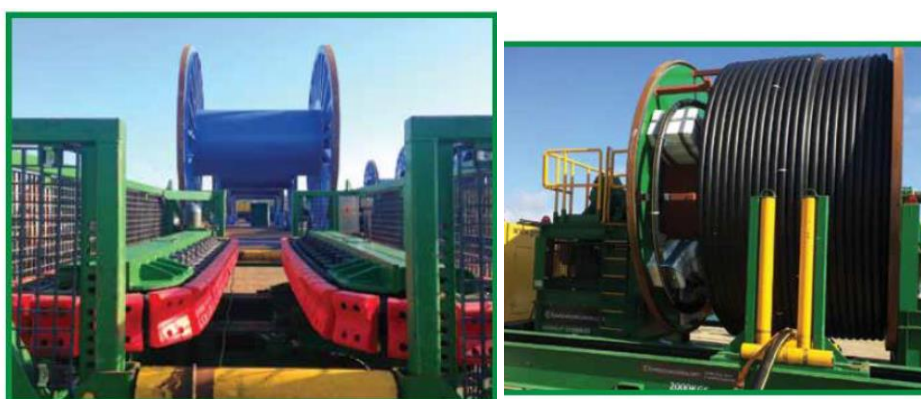
Figure 9: photos of the equipment used to unwind the export cable
