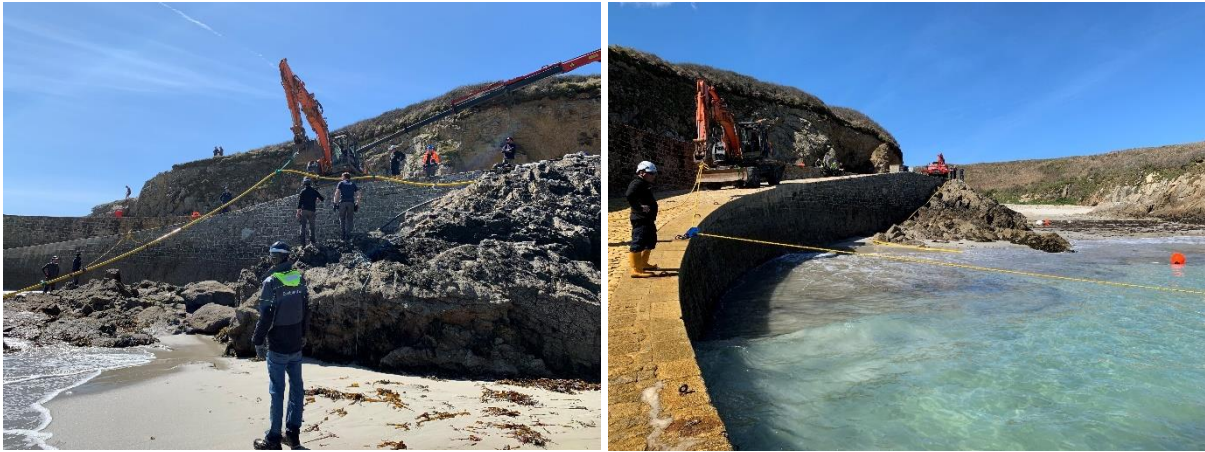
Figure 20 : repositioning the cable along the dyke and on the rock face
