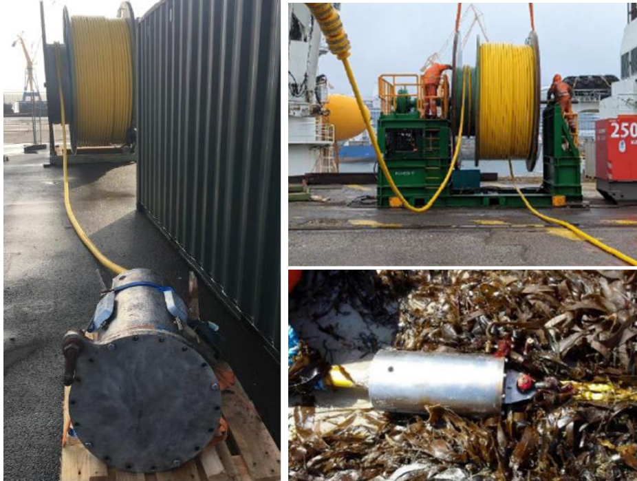
Figure 15: (left and top right) photos of the new export cable drum with both ends accessible and the dry-mate connector fitted beforehand, (bottom right) the abandonment head.
