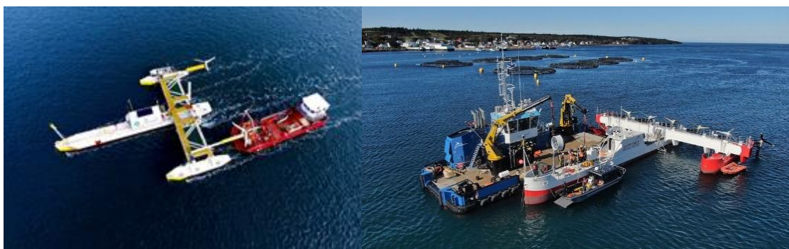
Figure 38 | Medium work boats for marine operations: PLAT-I blade change (left) and install (right)
