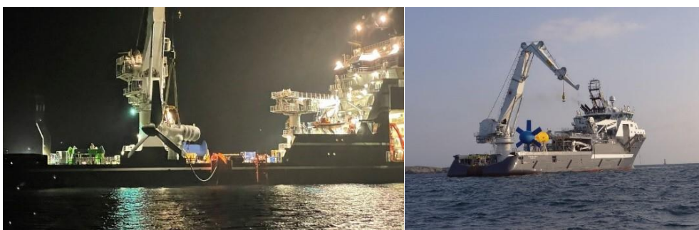
Figure 40 | Large vessel operations: AR500 (left), D10-1000 (right)
