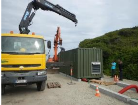
Figure 21: Installation of the conversion and control container (SABELLA SAS)
