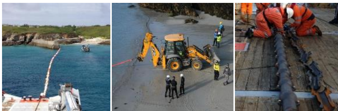
Figure 12: Positioning of the Argonaut - pulling the cable onto the beach - placing the shells (SABELLA)
