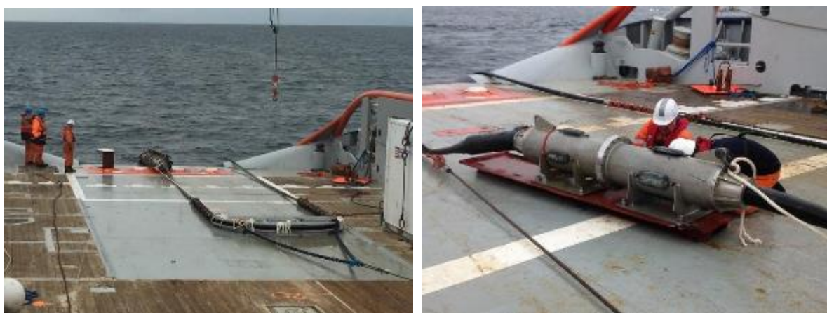
Figure 18: Connection of the tidal turbine to its electricity export cable - 21/09/2015 (SABELLA)
