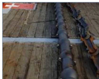
Figure 8: Composition of the export cable and shells installed on the cable in the hard substrate area (SABELLA)
