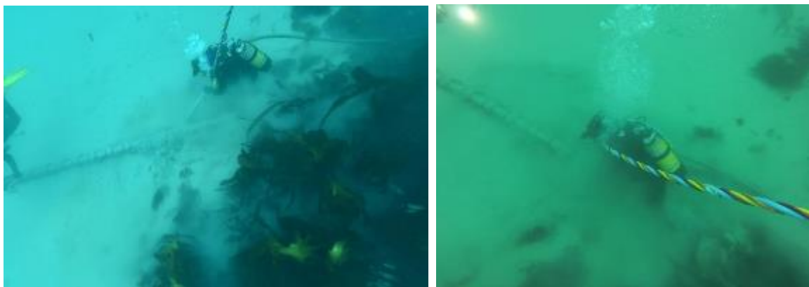
Figure 14: Embedding the cable in the sandy area (SABELLA)
