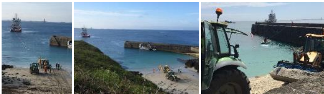
Figure 19: Means for installing the cable on the foreshore (SABELLA)
