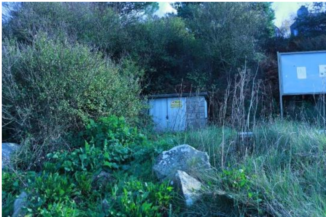
Figure 67: Lift station located at the top of the Tréno beach, Arzon (UBS, 2018)
